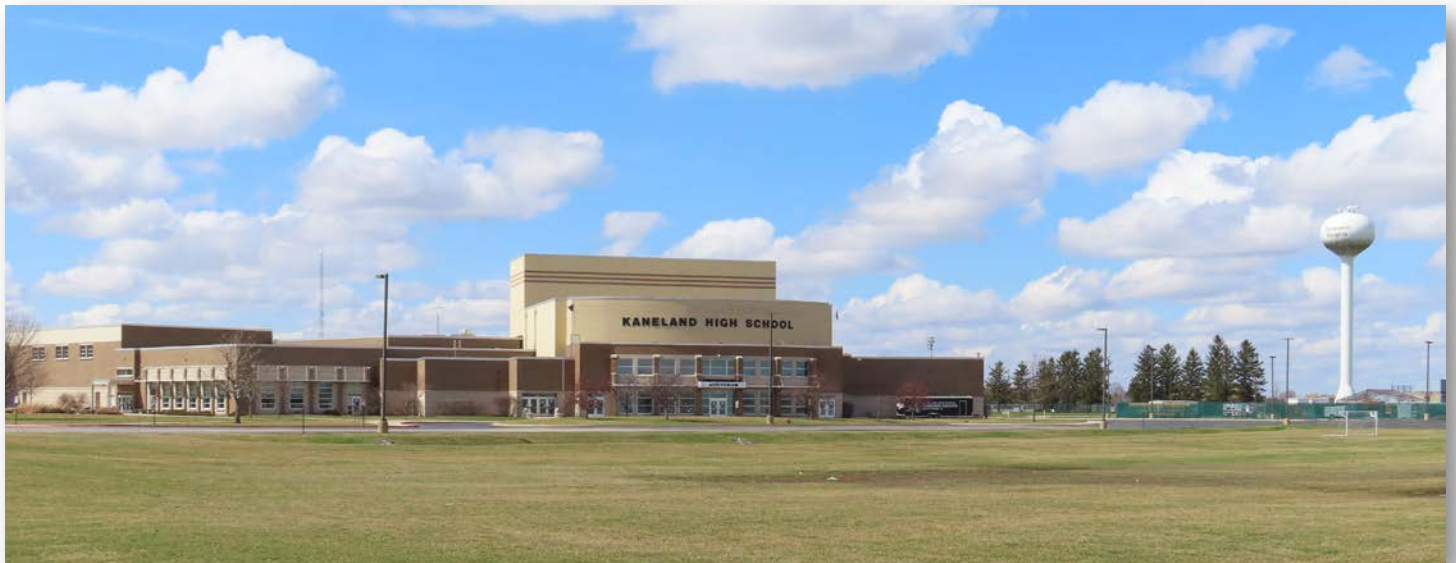
looking northwest from Keslinger Road, 4.120 Kaneland High School (across Meredith Road (east) from Feldott Farm)
