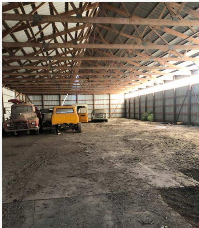
shed - 120' x 52.5' (all dirt floor)
